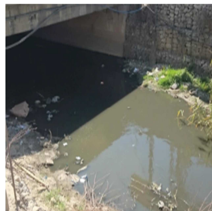
Figure 2. Site at Deir Zanoun.
